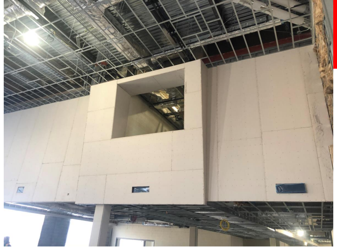
Gypsum Board Installed in New Addition Media Center
