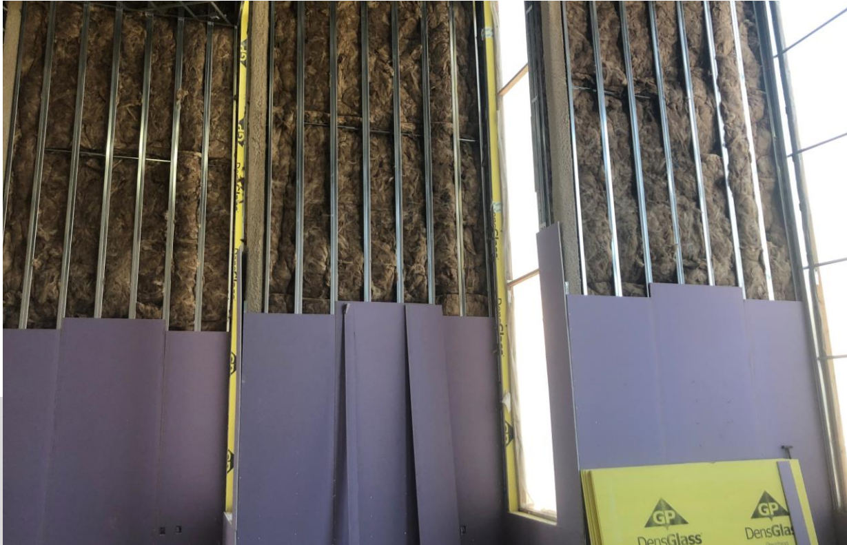
Installing High Impact Gypsum Board on Media Center Metal Stud Walls
